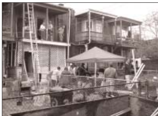
WTP making a difference on “Rebuilding Day.”
